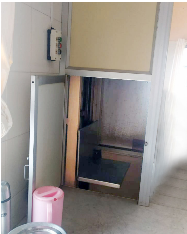
Food Lifting Machine Solar powered which carries food from the kitchen, Jeevan Jyothi Trust
