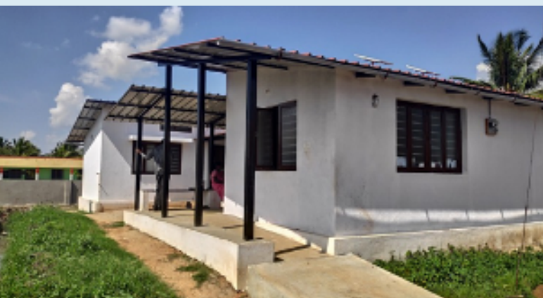
YK Mole Sub Centre designed to ensure thermal comfort for the patients and the health care staff, and reduce energy consumption; ANM Bhagya administering a patient at the YK Mole sub-centre, Gumballi, Karnataka.
