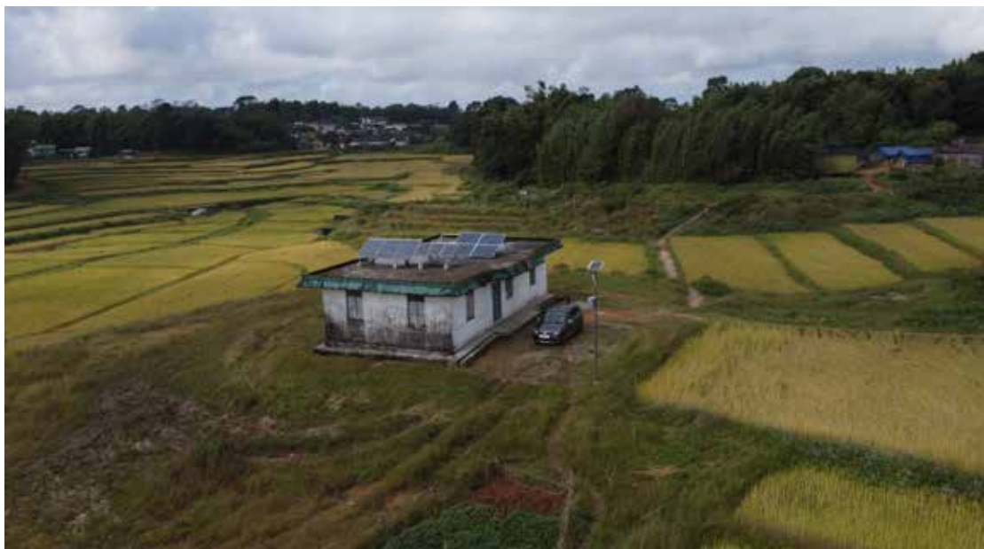
A solar powered sub center in Manipur
