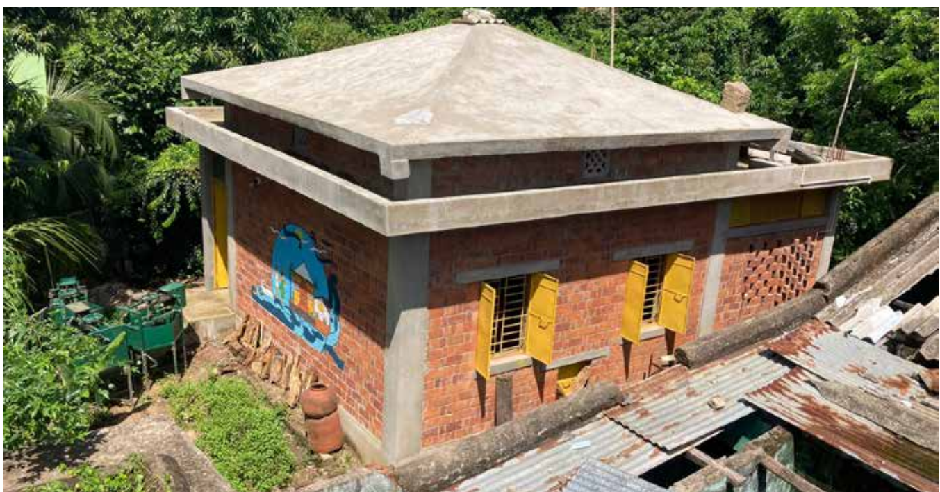
An efficiently built workspace for potters in cyclone prone regions
