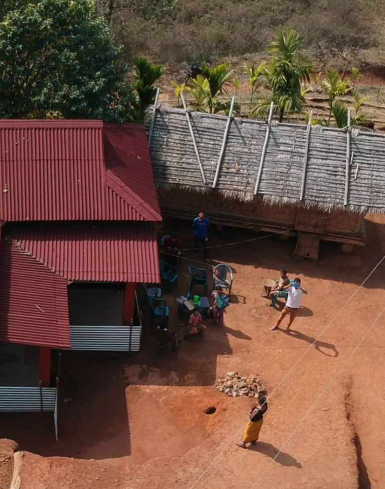
Aerial view of onduline roofing for a House in East Garo Hills, Meghalaya. Project done in partnership with DC Office, East Garo Hills
