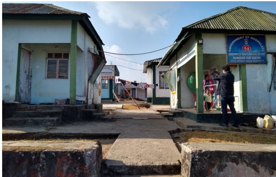
Figure 5: A solar-powered Health Sub Centre.
