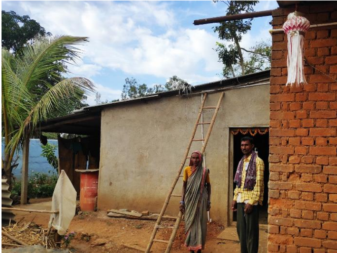
Before: Asbestos roofing, un-plastered walls and low ceilings resulting in dark and heated spaces
