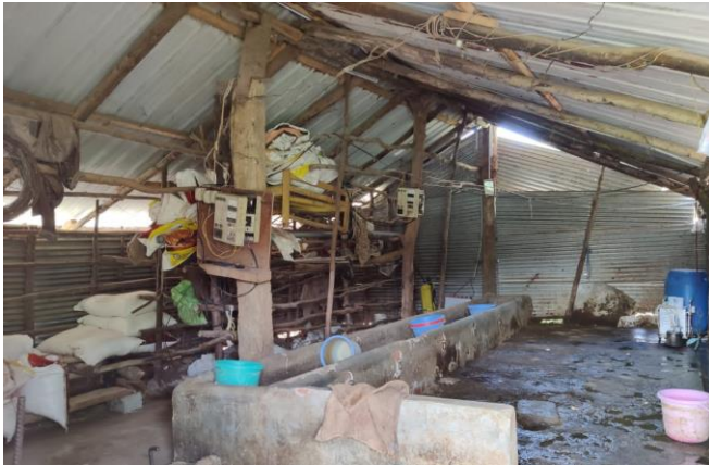
(Before) Ad-hoc built cow shed with thatch roof and tin sheet envelop
