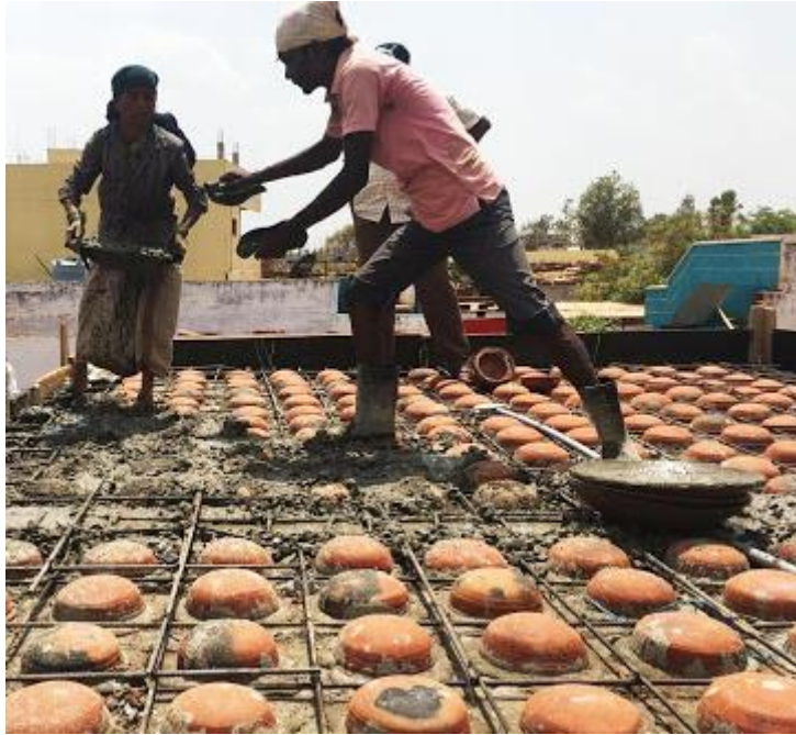
Seen: Construction of insulated RCC filler roof slabs
