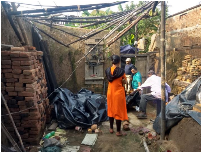
Before: Cyclone devastated workspaces
