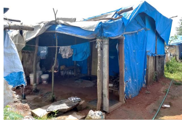
(Before) Blue tarpaulin sheet housing and flat pack tents get overheated in the afternoons
