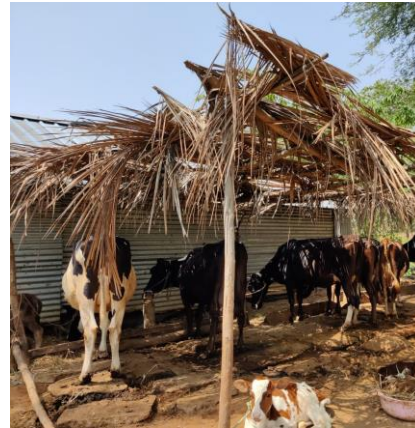
(Before) Ad-hoc built cow shed with thatch roof and tin sheet envelop
