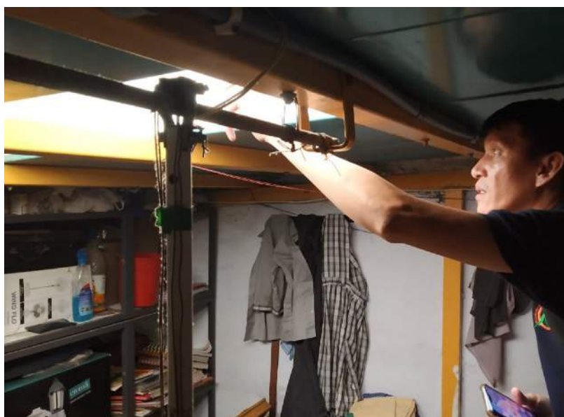
Member from Manila Housing Trust installing Energy Efficient Housing Solutions
