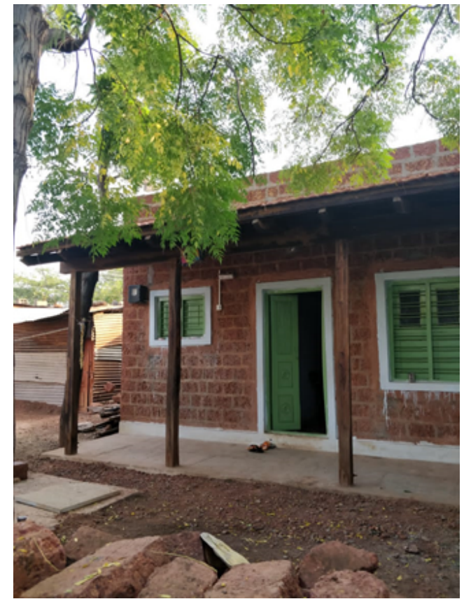
AFTER: Indoor Temperature was recorded 4°C lower than outdoor temperature. This has resulted in an over 10°C difference in the indoor temperature for the family from the older house to the new house.
